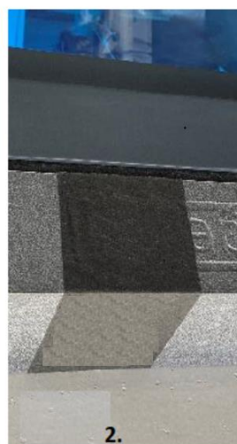
Additional sealing of joints of EPS profiles - with stretching windows foil
